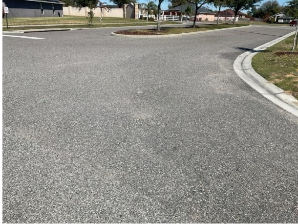
Pavement overview at Fillmore Boulevard
