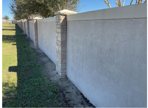
Concrete perimeter wall overview
