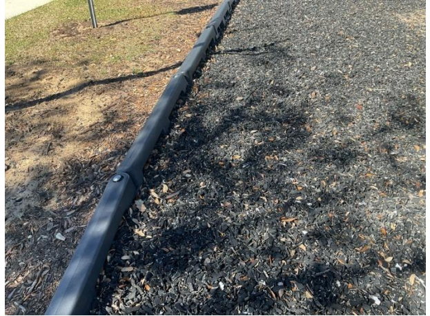
Safety surface and border at Citrus Isle
