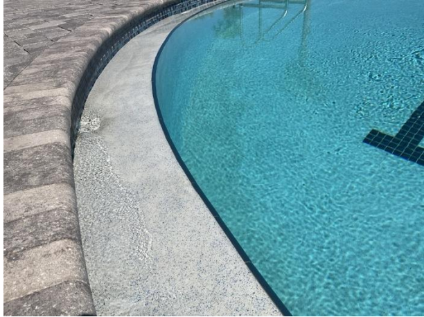
Pool plaster finish with tile perimeter
