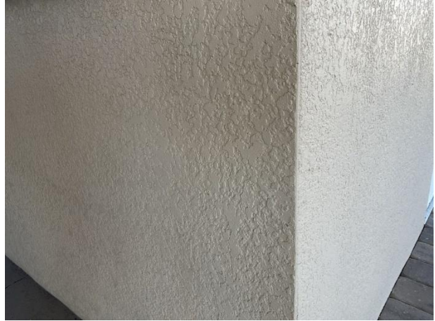
Stucco wall finishes
