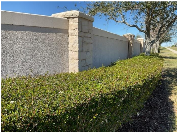
Concrete perimeter wall overview
