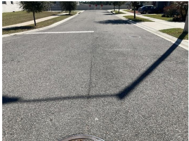
Pavement overview at Buchanan Drive
