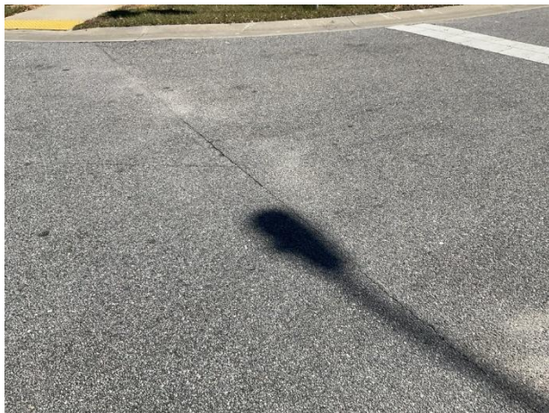
Pavement cracks
