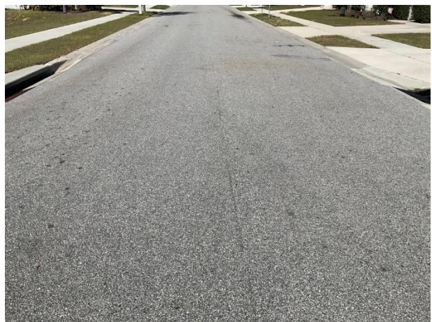
Pavement overview at Jefferson Street
