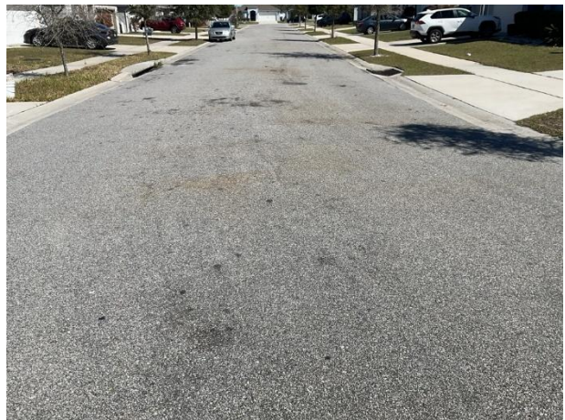
Pavement overview at Fillmore Court
