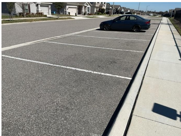
Pavement overview at Citrus Point pool area
