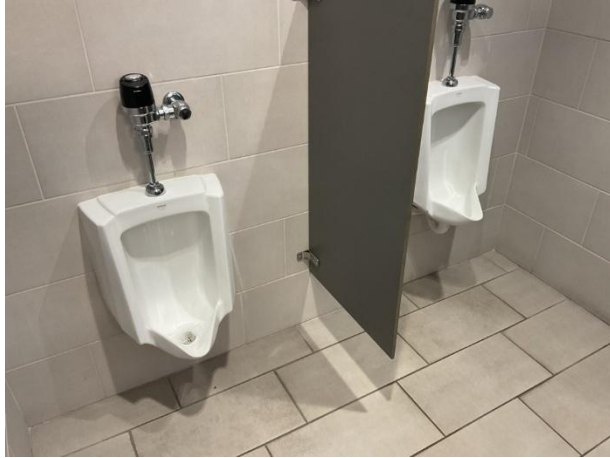
Rest room overview
