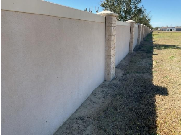
Concrete perimeter wall overview
