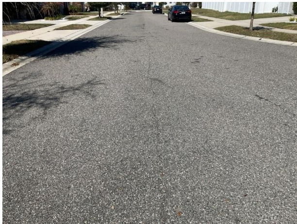
Pavement overview at Buchanan Drive
