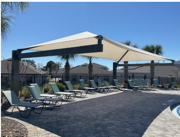
Shade structure overview
