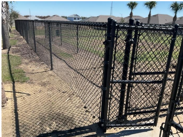
Chain link fence
