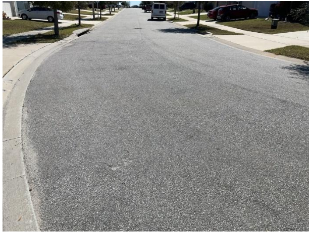
Pavement overview at Taft Drive
