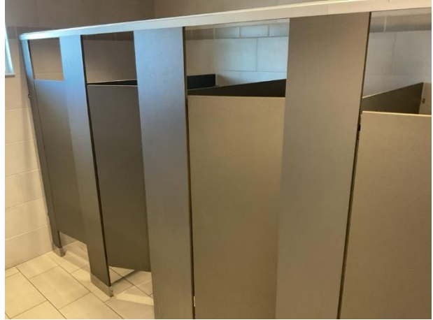
Rest room overview
