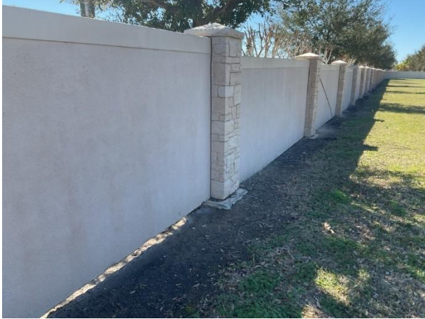
Concrete perimeter wall overview
