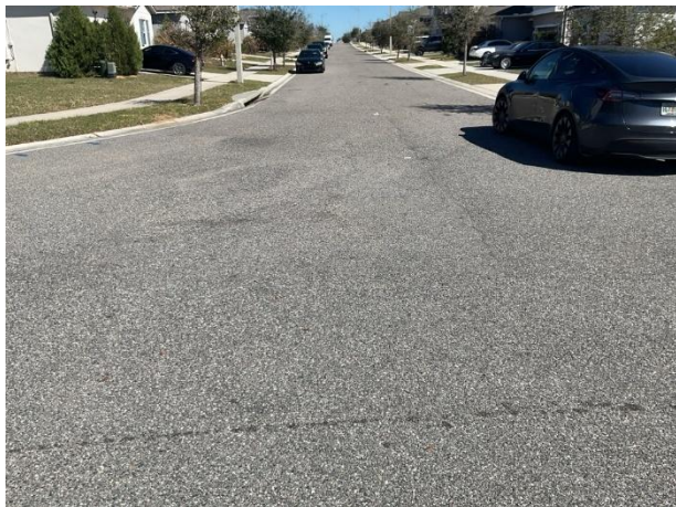
Pavement overview at Buchanan Drive
