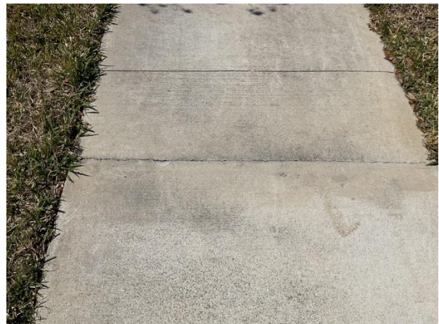
Sidewalk cracks
