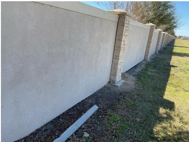
Concrete perimeter wall overview
