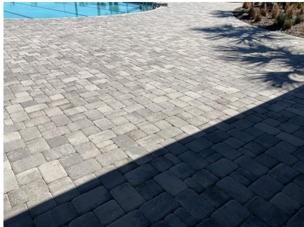
Paver pool deck overview
