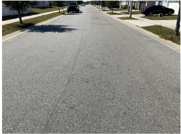
Pavement overview at Taft Drive
