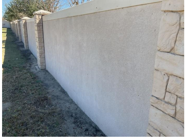
Concrete perimeter wall overview
