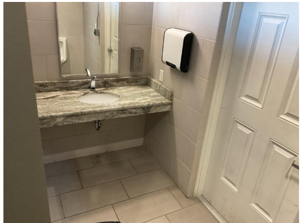
Rest room overview
