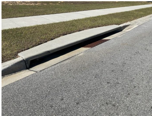
Typical catch basin
