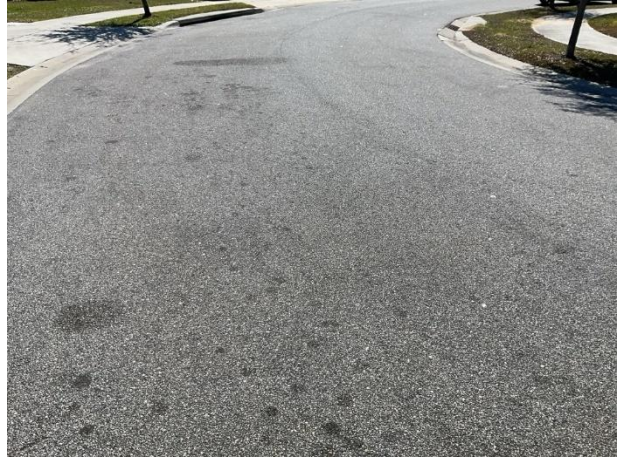
Pavement overview at Taft Drive
