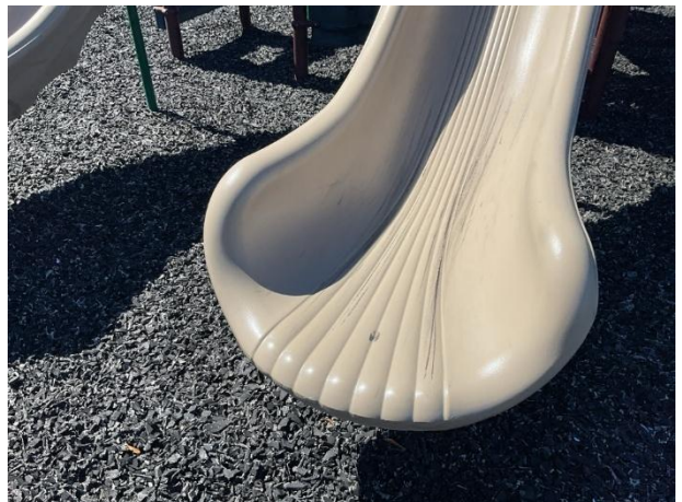
Equipment finish deterioration
