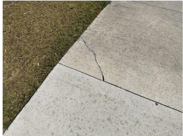
Sidewalk cracks
