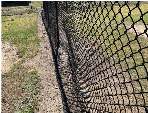
Fence warped webbing
