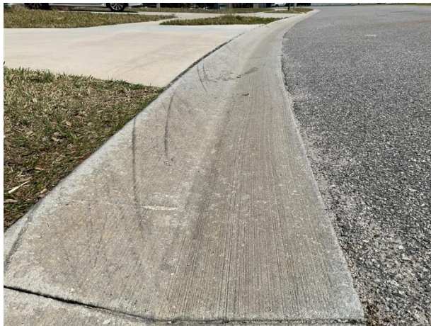
Concrete gutter overview
