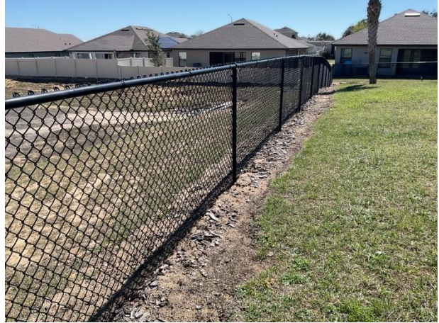
Chain link fence
