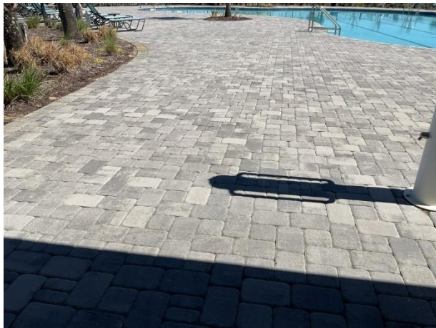
Paver pool deck overview
