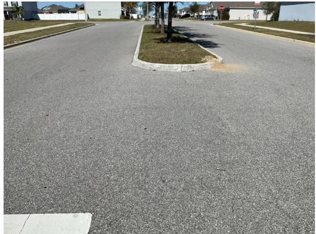
Pavement overview at Jefferson Street
