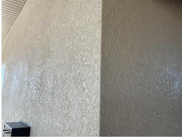
Stucco wall finishes
