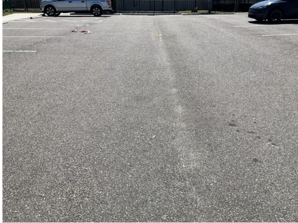
Pavement overview at Citrus Point pool
